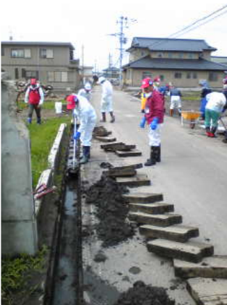
Cleaning the street gutters
